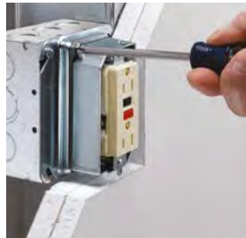
03 Re-tighten... Adjustment screws.
