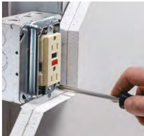
01 Loosen... The two adjustment screws located on opposing corners of the mud ring.
