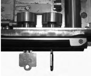
Key Interlock Facility
