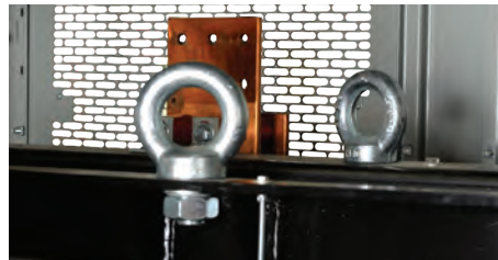
Lifting eyes for core & coil assembly
