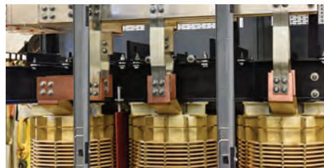
Low voltage bus bar
