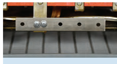
Expanded neutral bar for multiple customer connections
