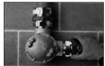
6. Insert cable and tighten red union
