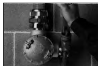
5. Install hub on enclosure
