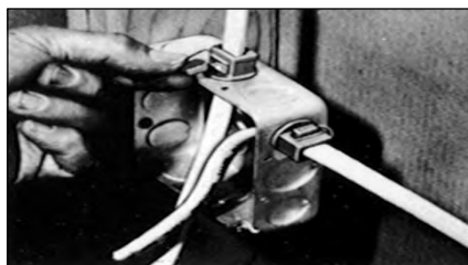
Snap captive locking wedge into connector's cavity.
