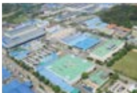
Cheongju Factory (Korea) Electric Products, Mold TR, MV/LV Switchgear, and HV GIS
