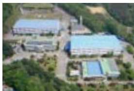
Cheonan Factory (Korea) PLC, AC Drive, HMI, DCS, and PV Module
