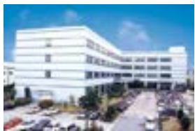
Power Device R&D Center Leading technology in electric industry and continuously developing future-growth dynamic engines
