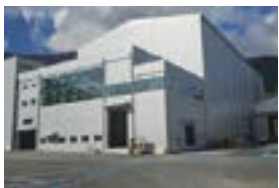
Ulsan Factory (Korea, LS Power Solution) HV TR, Mold TR, and Pad TR
