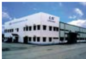
Hanoi Factory (Vietnam) MV/LV Switchgear, and Mold TR
