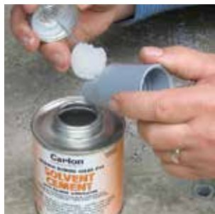
Apply a uniform coat of cement.
