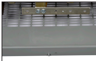
Bottom cable entry area where applicable
