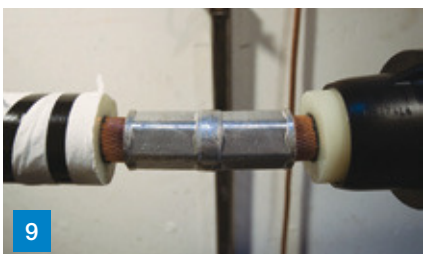
9 Conductors shown joined using a compression connector.
