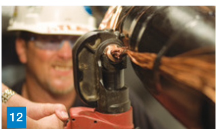
12 Connect neutral wires as required.
