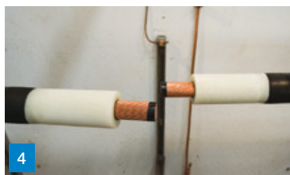
4 Bare the conductor.
