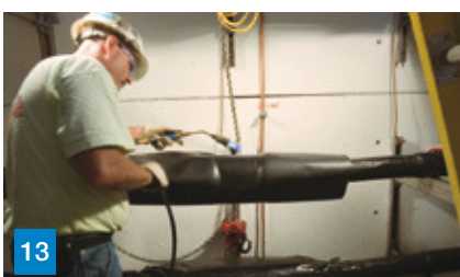
13 Position and shrink cover-ups.
