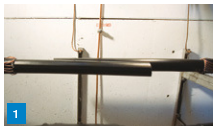
1 Overlap cables, straighten and strip back jacket.
