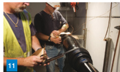
11 Seal joint ends with mastic wrap.
