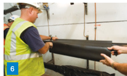
6 Store the cover-up sleeve on each cable.
