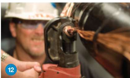
12 Connect neutral wires as required.
