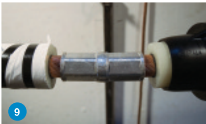
9 Conductors shown joined using a compression connector.
