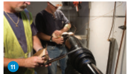
11 Seal joint ends with mastic wrap.
