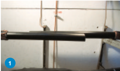
1 Overlap cables, straighten and strip back jacket.
