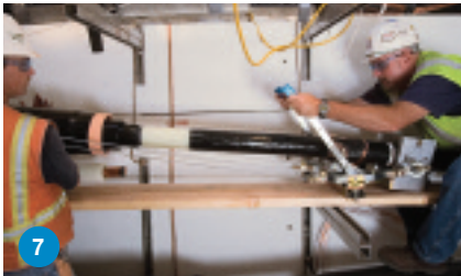
7 Pull TCJ joint housing into the storage position on the cable.
