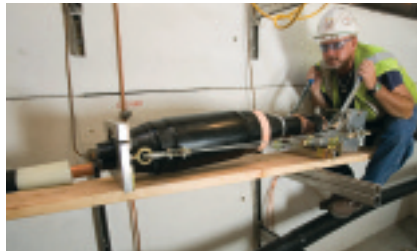
7 Pull TCJ joint housing into the storage position on the cable.
