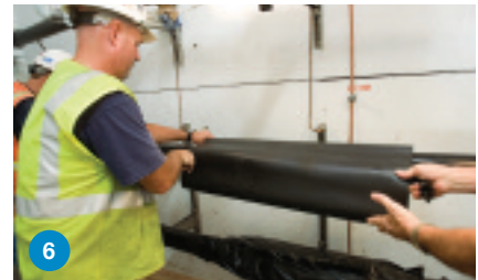
6 Store the cover-up sleeve on each cable.
