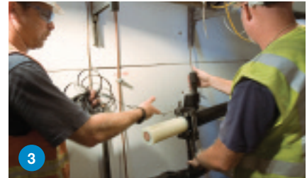
3 Remove the semi-conductive shield...
