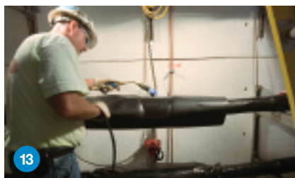
13 Position and shrink cover-ups.
