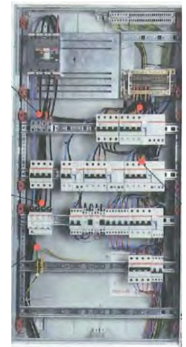
Conventional DIN rail assembly
