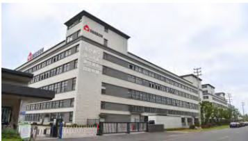
High-tech zone site
